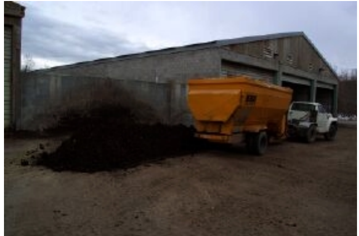
Mixing sewage sludge and sawdust for static pile composting at the Hoosac Water Quality facility in Williamstown, MA.
