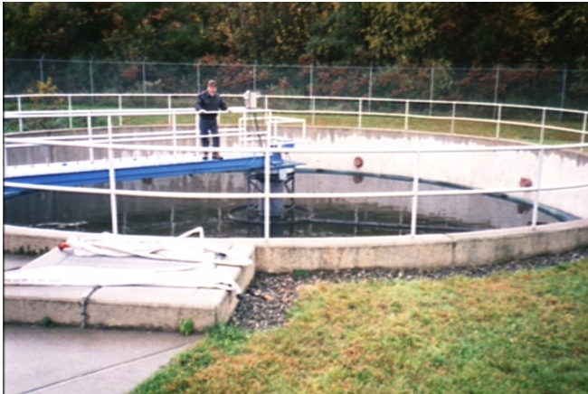
A secondary clarifier at the Windsor, VT, WWTF. Clarifiers mimic the conditions in a still pond, allowing solids to settle to the bottom where they are removed by a slowly-rotating scraper. These solids are then treated to become biosolids.
